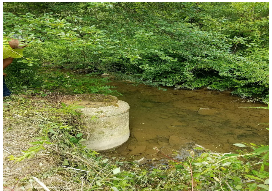
Manhole Located in Stream (Scholars Run Interceptor)
