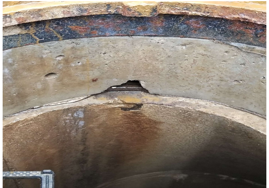
Cracked Manhole
