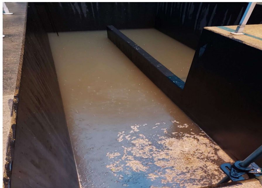
Chlorine Contact Tank – solids in tank
