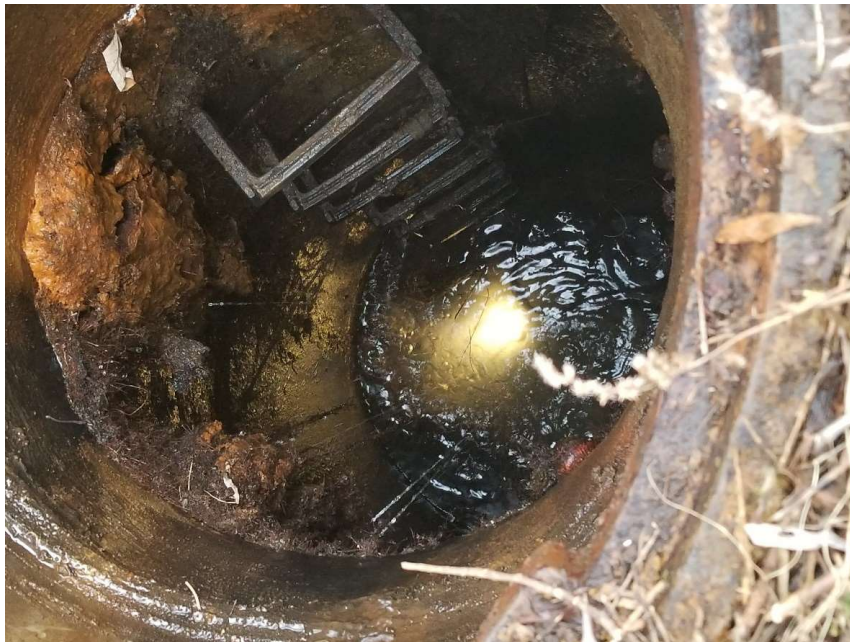
Surcharged Manhole - Roots
